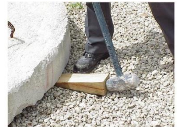
Inserting a wedge to initiate cribbing
